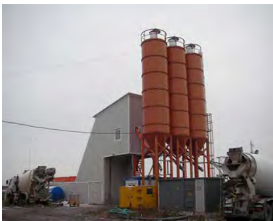
SC EUROCONSTRUCT SRL, SMIS 56769
